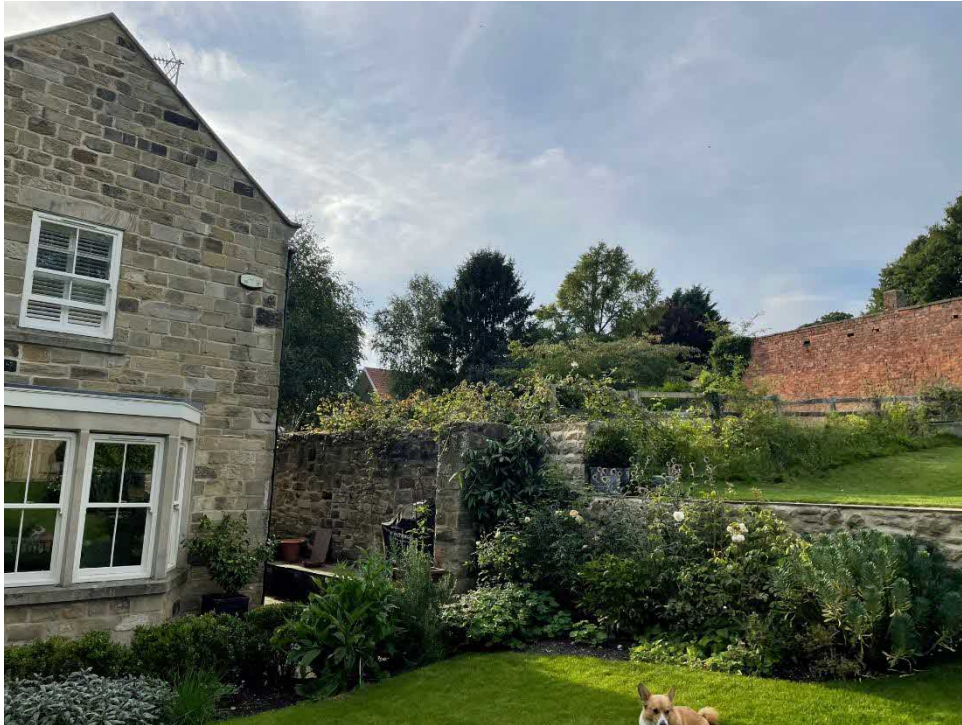
Rear elevation to 1 Manor Court showing change in levels
