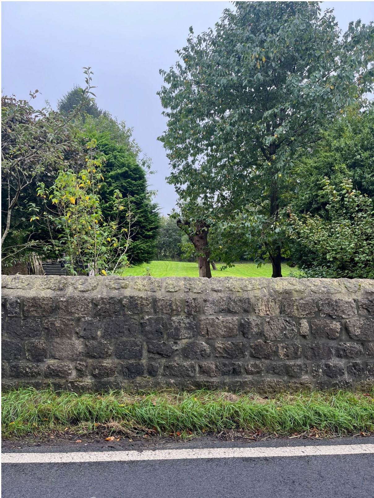
Image: View Looking South from Stang Lane into the Area of Important Open Space adjoining the Old Crown. Evidently, the site has an unambiguous street frontage with views possible across the site.
